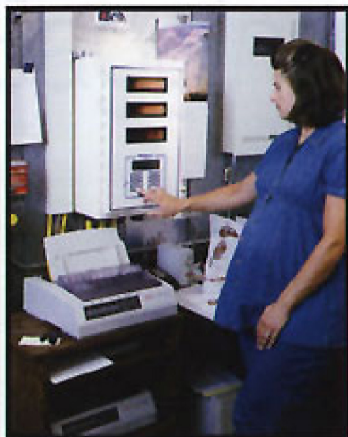
PLC-based control system can load 100 recipes, which can be run by merely entering the recipe number on the operator panel.
